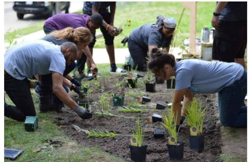
Volunteers with Clean Wisconsin install a rain garden in Milwaukee [16]
