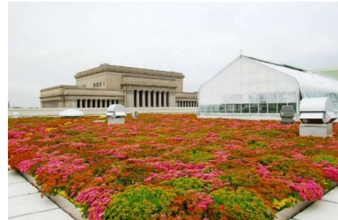
Green roof at Milwaukee Public Museum [14]
