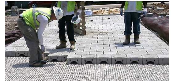
A cross view of PavDrain® pavers [12]
