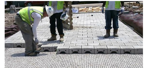
A cross view of PavDrain® pavers [12]
